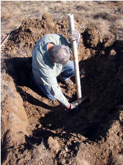
Photo 3 (below): The 2-inch PVC casing, for each monitoring well to be abandoned, was cut off 24 inches below ground surface.
