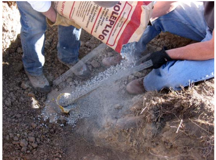
Photo 3 (below): The 2-inch PVC casing, for each monitoring well to be abandoned, was cut off 24 inches below ground surface.
